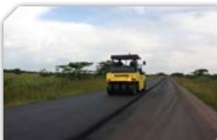
Asphalt Overlay Kawempe-Kafu Road
