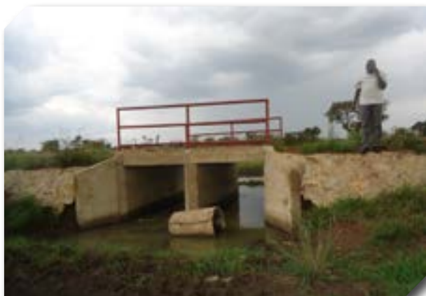
Figure 10.1: Box Culverts constructed along Abalanga – Agonga Road in Amuria District
