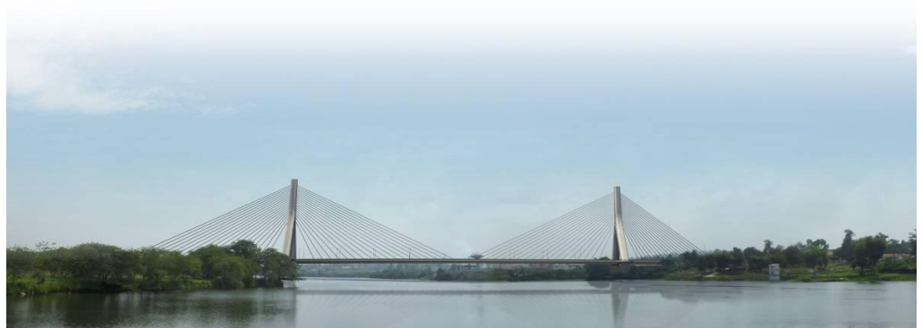
Cable-stayed design for Second Nile Bridge at Jinja
