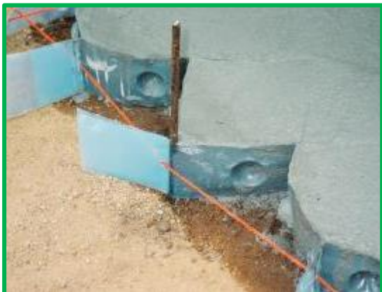
Geocells during construction
