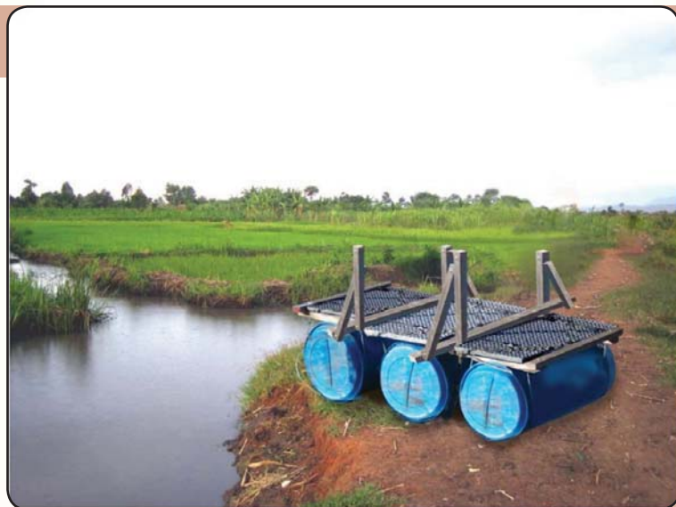
Construct timber deck on top of the plastic drum assembly to form a platoon. Several platoons are made sufficient to bridge the water crossing area.
