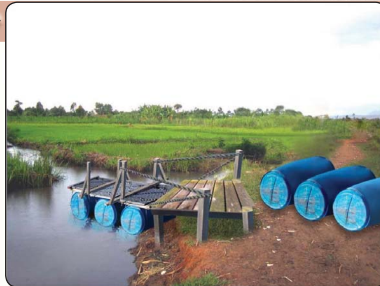
Landing deck constructed and joining of 1st platoon to the landing deck using ropes starts.
