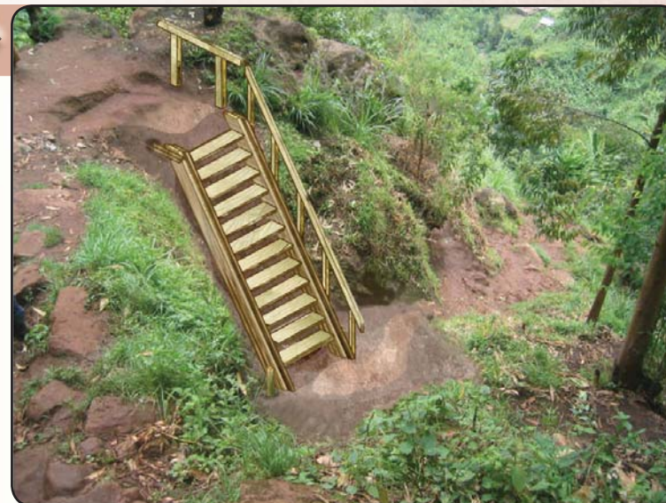
Ladder assembly complete with handrails ready for use.
