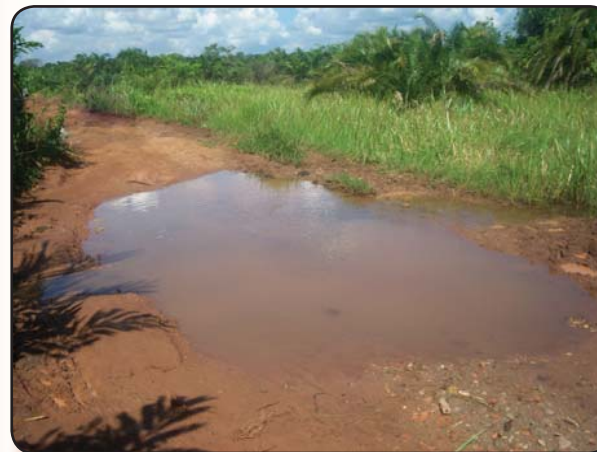
The picture shows water crossing at the surface of the access road
