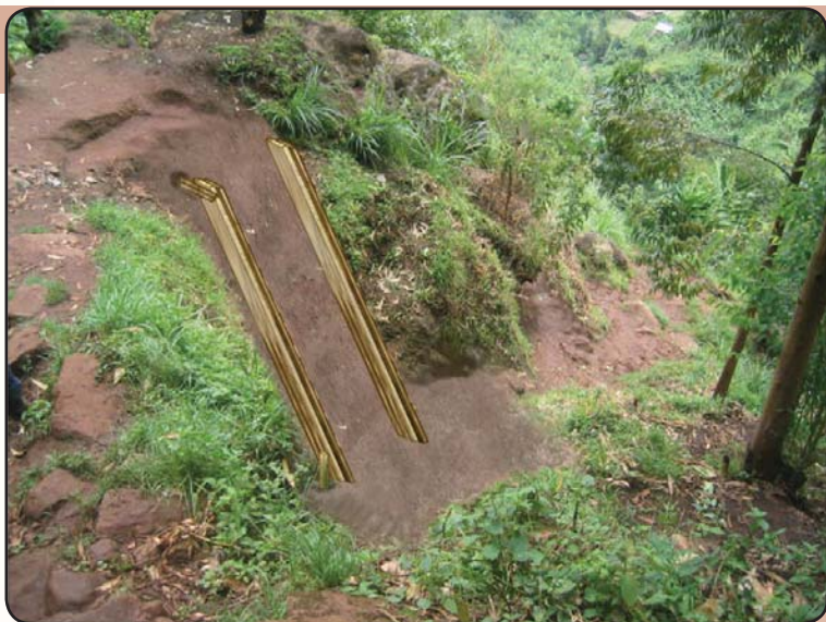
Install ladder footings into foundation using class 20 concrete. After 28days ladder assembly begins.
