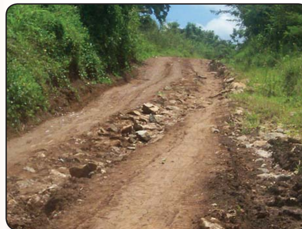
A deteriorated gullied section of a community access road.
