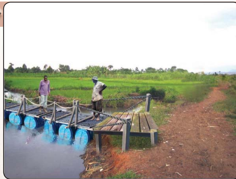
The remaining platoons are joined in succession until the whole bridge is completed ready for use.
