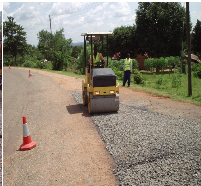
Fig-9: Rolling over 20/40 stone with 1.7 t roller
