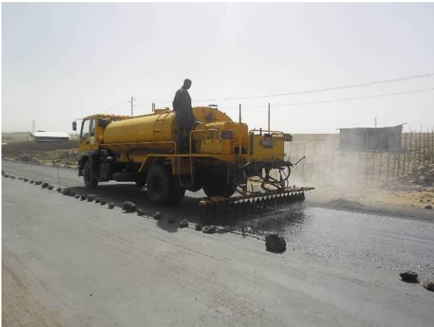
Figure 3 Bitumen spraying
