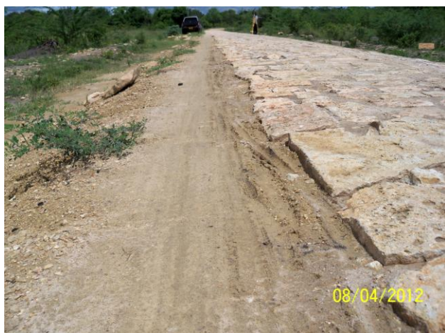
Figure 6 - Hand Packed Stone Shoulder Wear
