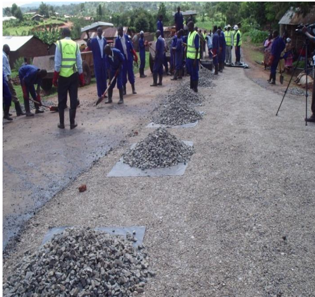
Fig-6: Spotting of 20/40mm stone
