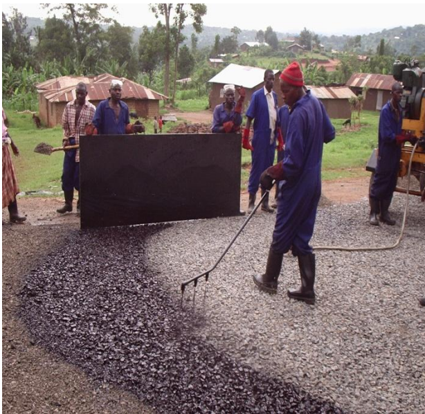
Fig-8: Applying the 2.9 l/m 2 as 1 st penetration
