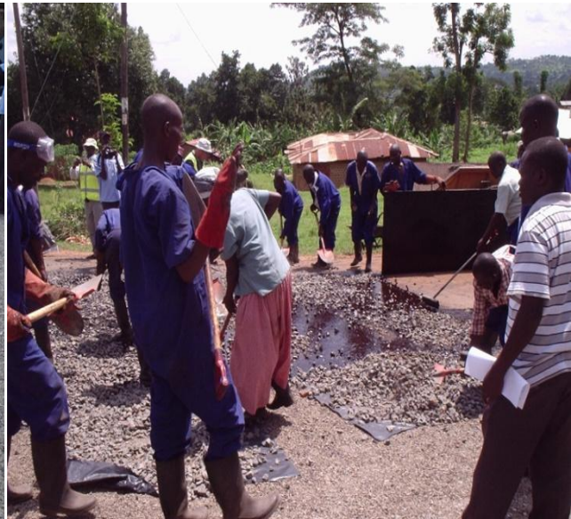
Fig-7: Laying 20/40 stone on tack coat
