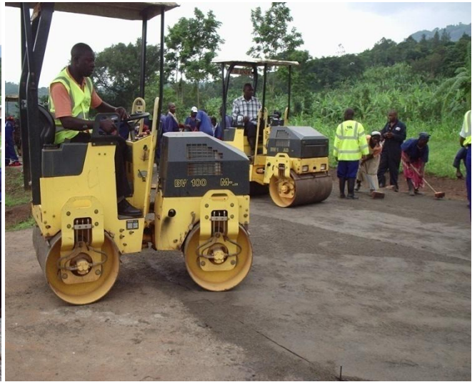
Fig-11: Rolling sand with 1.7 t sit-on rollers
