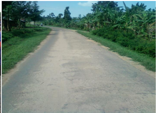
Fig-13: Completed sand seal section
