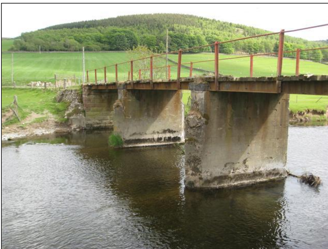
Figure 4: Dilapidated composite bridge at Easter Dawyck, Peeblesshire, Scotland.
