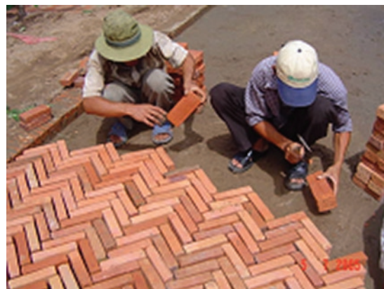
Photo 8: Laying burnt clay brick paving
