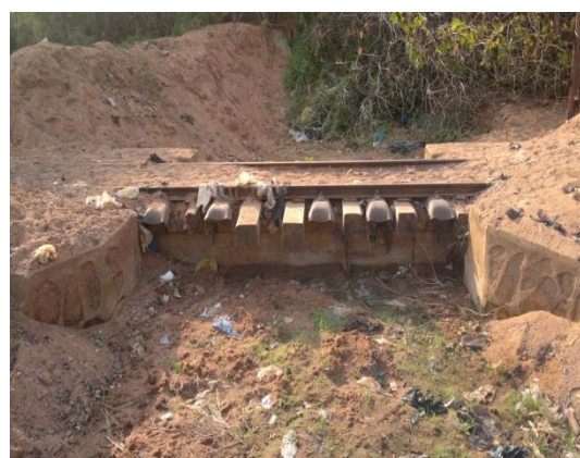
Figure 54: Blocked culverts at the Kigoma station yard
