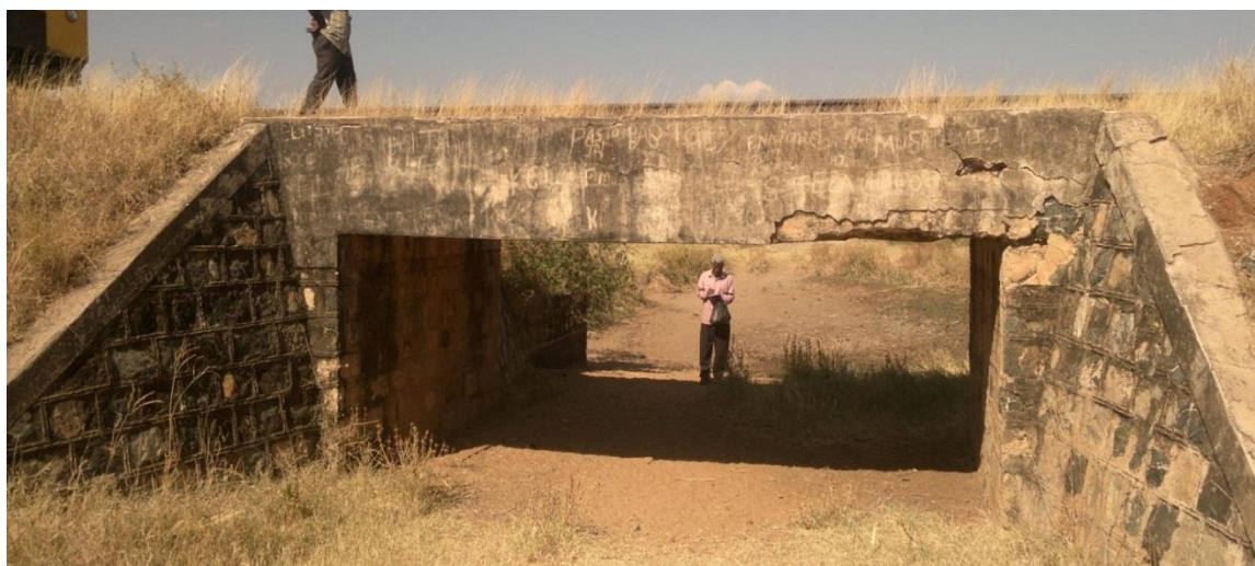
Figure 42 Typical German bridges Steel beams encased in concrete deck supported by stone masonry abutments
