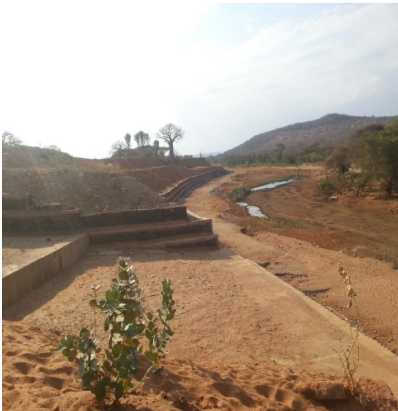
Figure 41 River bank protection Mkondoa River between Kilosa and Gulwe
