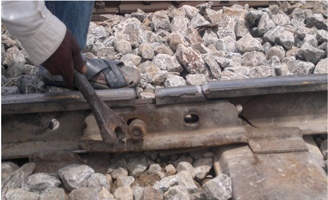
Figure 38 Worn out and Broken 56.12lb/yd rail ends and joint fittings
