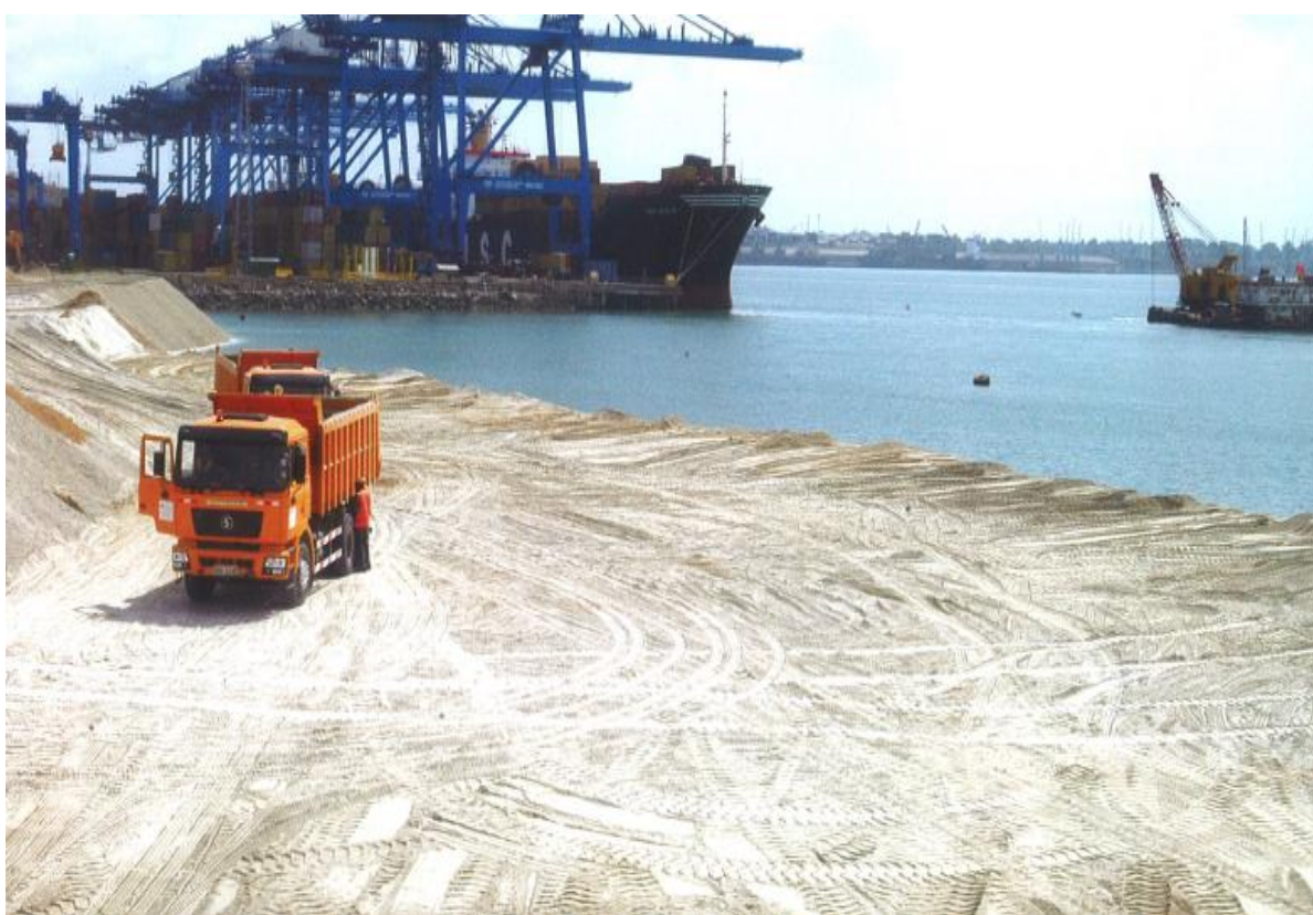
Figure 5: Land reclamation works for the Berth 19 project (Bandari 12/2011)
